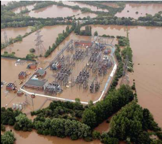
Castle Meads electricity substation flooded in 2007 leaving 42,000 people without power
