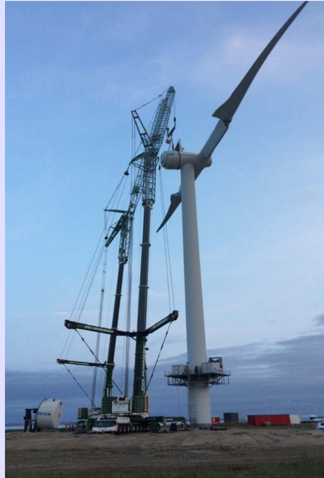
Lifting onto the Envision turbine
