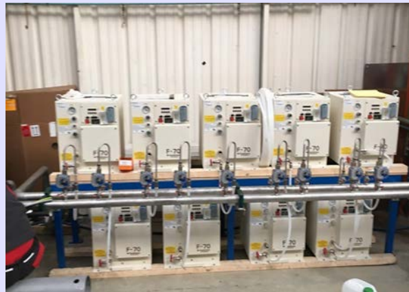
GM cold-heads & compressors
