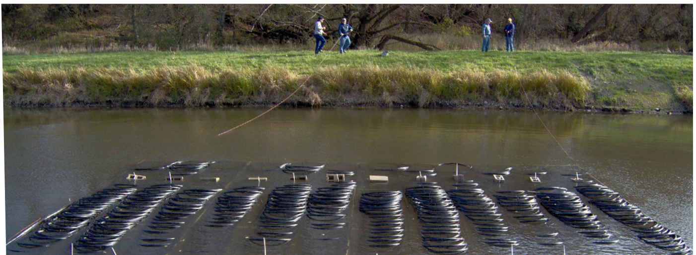
Figure 4: Water-source heat exchanger being installed By Mark Johnson (Markij at English Wikipedia) - Own work, Public Domain, https://commons.wikimedia.org/w/index.php?curid=7952259
